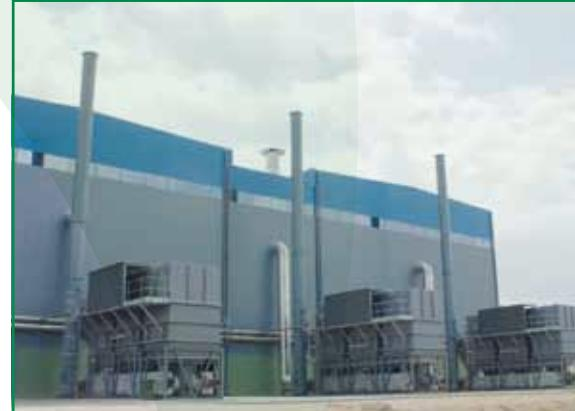
Primary and secondary heat recovery will be used wherever practicable and if the correct solution is a thermal oxidiser then this can sometimes be designed to operate in autothermal flameless mode, without the use of primary fuel.
